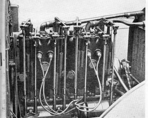
TWELVE CYLINDERS were used in the 1922 2-litre Delage which was world champion when supercharged in 1925, The exhaust manifold was in the "V" between the blocks.
