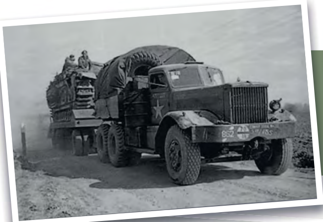
LEFT: In the Western Desert BELOW LEFT: The photograph that started this story. Sapper Brian Dean with a soft top 980/981, somewhere in the Western Desert MIDDLE LEFT: The left side of the engine gives an idea of the sheer bulk MIDDLE RIGHT: The right side of the Hercules DFXX six cylinder diesel engine
