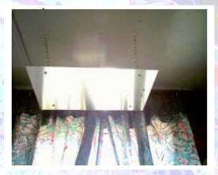
Next are the eye bolts, first place nut all the way up threads, then a flat washer, now push eye bolt thru SS sheet, on back side place another flat washer and nut. Ready? Tighten the nut you placed first, down to the SS sheet and snug the nuts up against each other, leaving the bolt just going past bottom nut to make a neat appearance. Repeat three more times.
