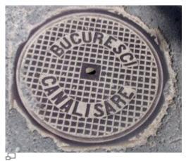
An old <u>manhole cover</u> in Bucharest, writing "Bucharest - sewerage" using etymological spelling, *Bucuresci - Canalisare* instead of *Bucureşti - Canalizare*
