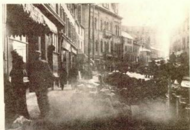
YESTERDAY: This 1899 photograph is a view of Main Street looking toward City Square from the corner of Winthrop and Main Streets. The tracks for the Boston Elevated Railway are shown under construction along Main Street.
