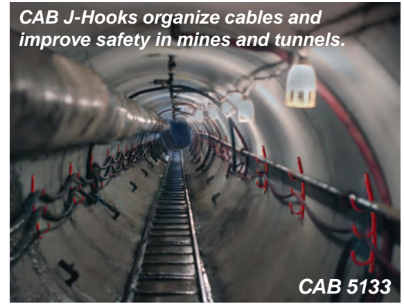
Multi-Carrier Hangers safely separate and support heavy cables. Custom sizes available.
