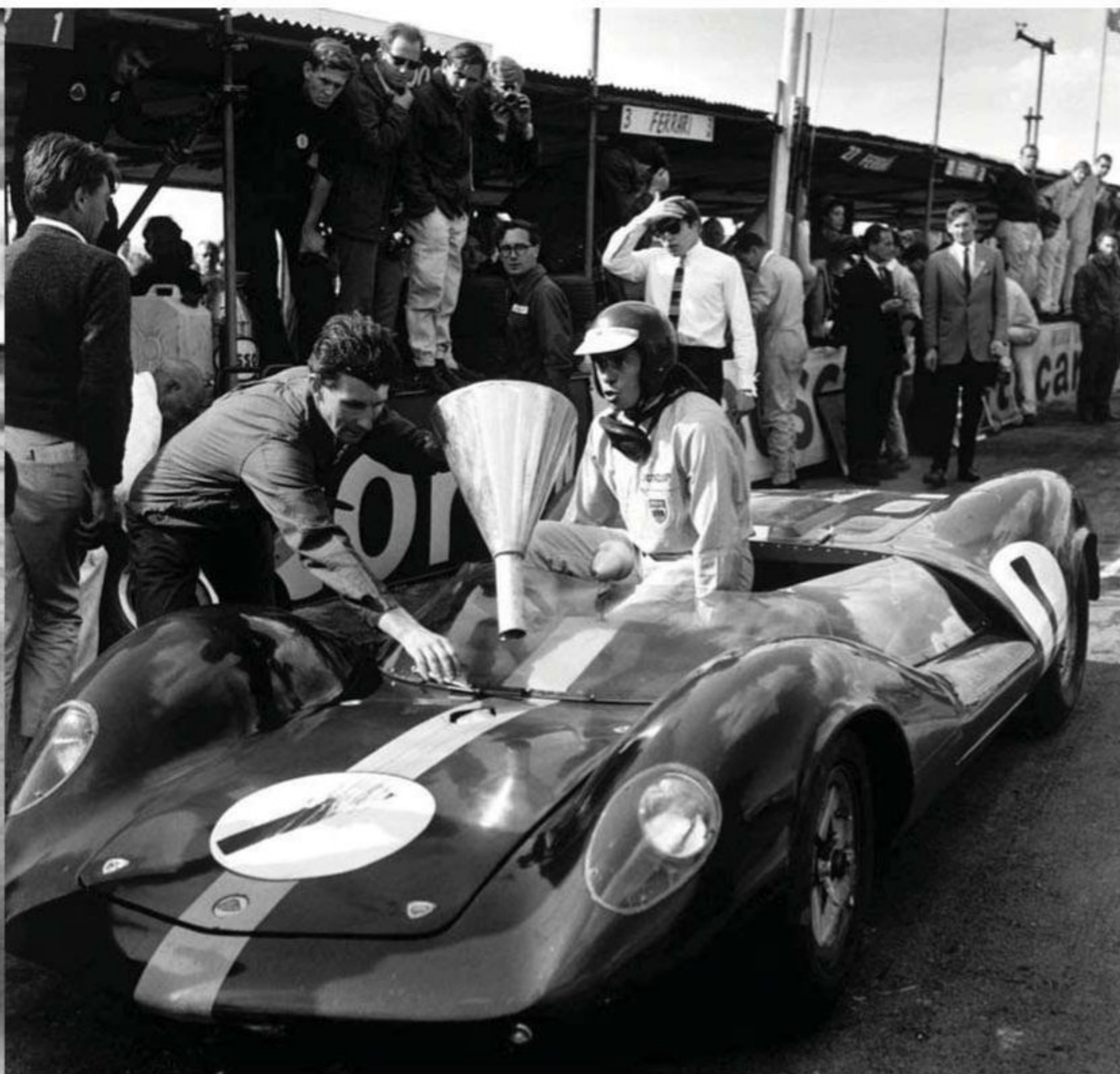
Features like the central fuel filler and one-piece body were clearly not thought out and often changed by customers
