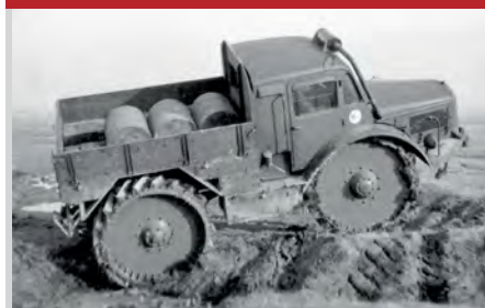
With deep cleats the big tractor made short shrift of most of its trial challenges, here with a simulated heavy load
