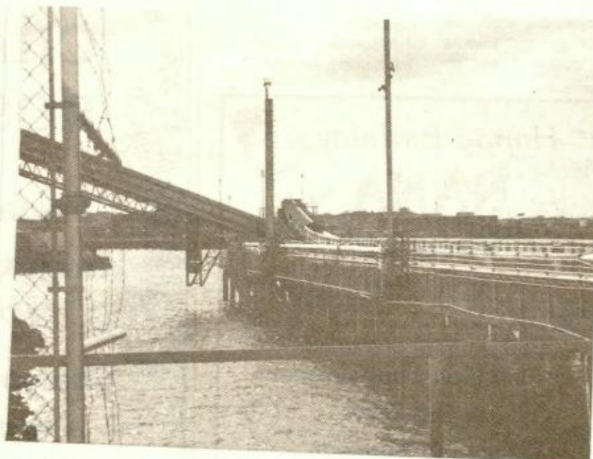
Street includes the crane, pier, dock and sugar storage facility. (photos by Lynn Peters)
