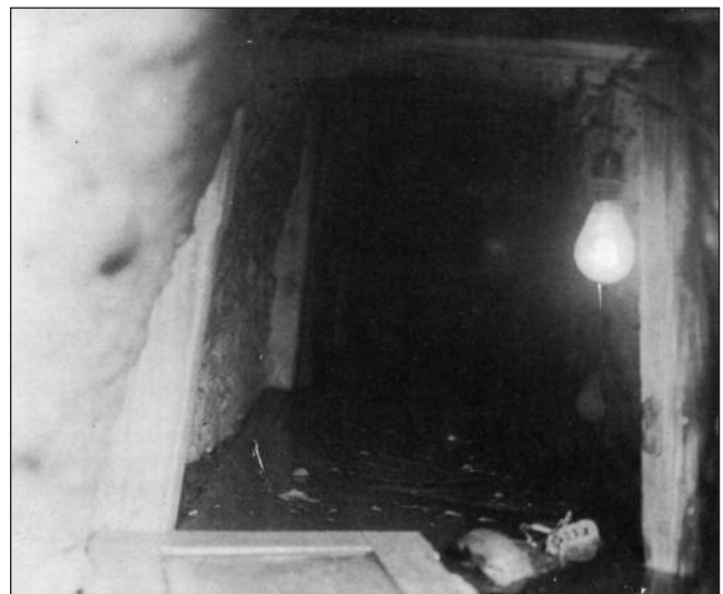
The house lay inside the wire, the tunnel emerging in the narrow path in the foreground. Above left and right: The tunnel, ten feet underground, was shored up with timber and lit with electric light.
