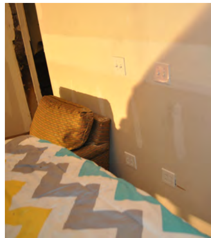
(b) Stud Cavity Electrical Installation
