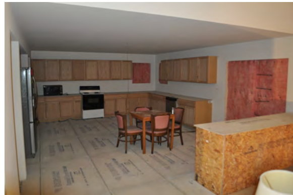
(b) Two Story Kitchen
