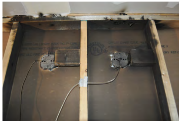
(e) Single Switch & Outlet Rear Top
