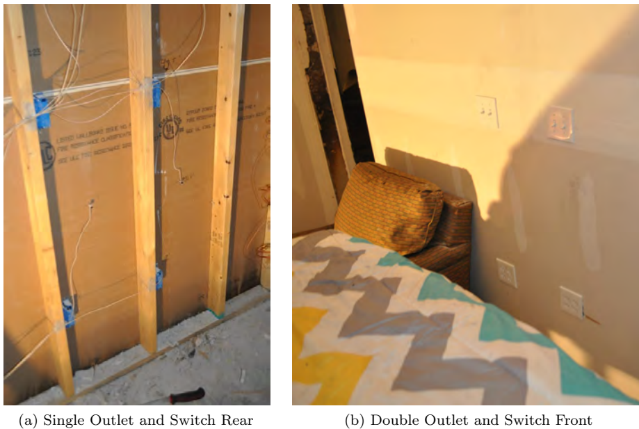
Figure 10.37: Void Space Wall Penetrations
