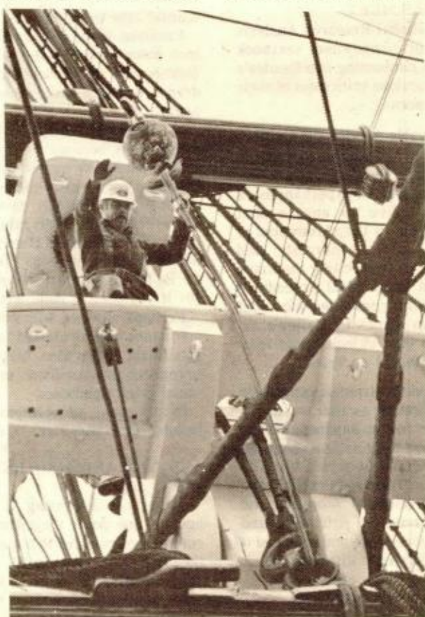
REPAIR WORK ON THE OLD IRONSIDES Gerald McCarthy of the USS Constitution Maintenance and Repair Facility, located in the Charlestown, Mass., National Historical Park, keeps a wary eye on the main yardarm of the USS Constitution as it is raised into its resting place after restoration efforts. (U.S. Navy photo by J02 James P. Woodworth)
