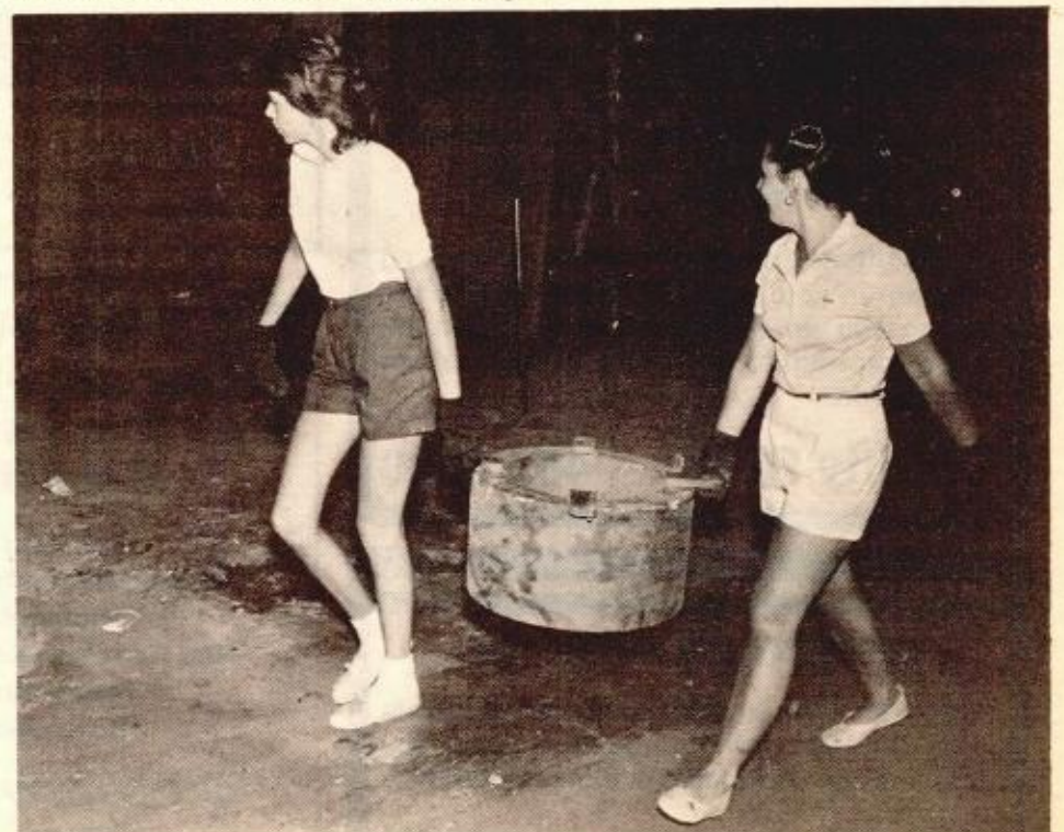
TWO CHARLESTOWN GIRLS carry one of the wooden patterns from Building 104. It was agreed between the Boys and Girls Club and the Artists Foundation to split in
