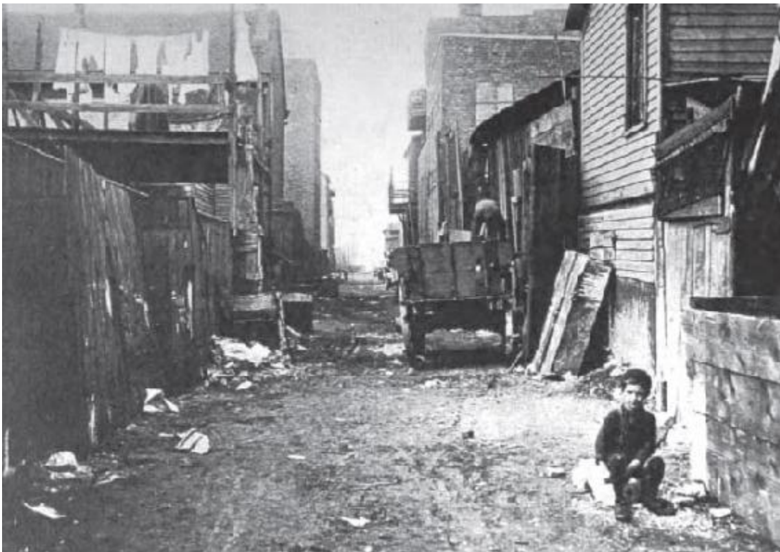
Photo 1.4: The general insanitary conditions which surround the houses on both sides of the alley. The first house on the right is a small dilapidated frame house. Beyond it are three larger tenements. The outbuildings at the left are all dilapidated, and contain privies which are in a foul condition. There are not
