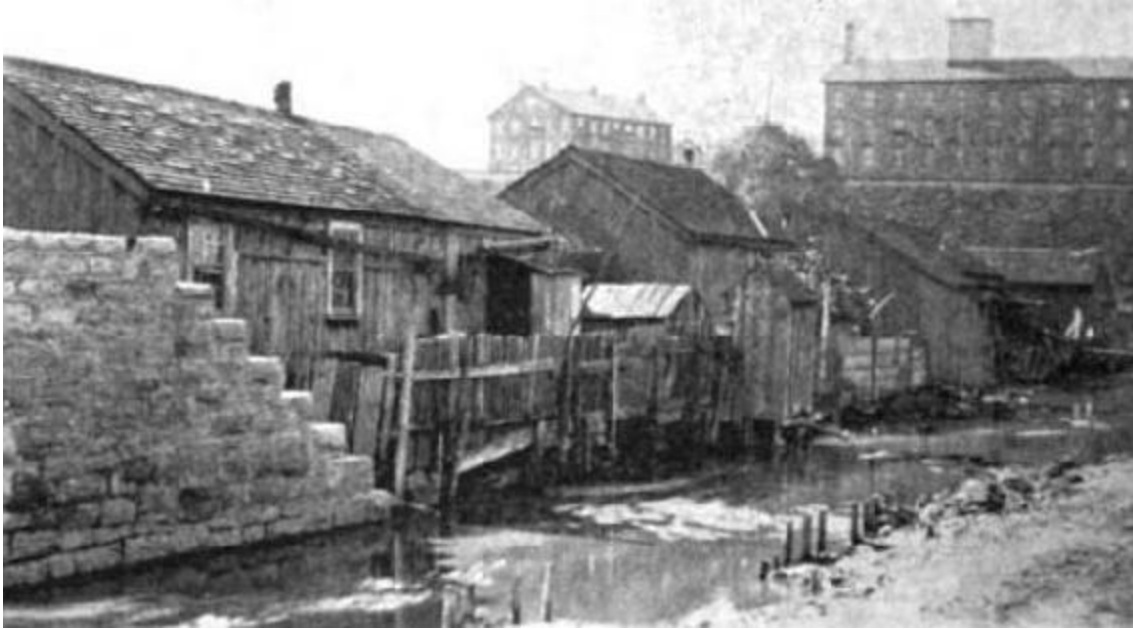
Photo 1.1: Syracuse, NY—Shanties Back to an Open Sewer. (1901)
