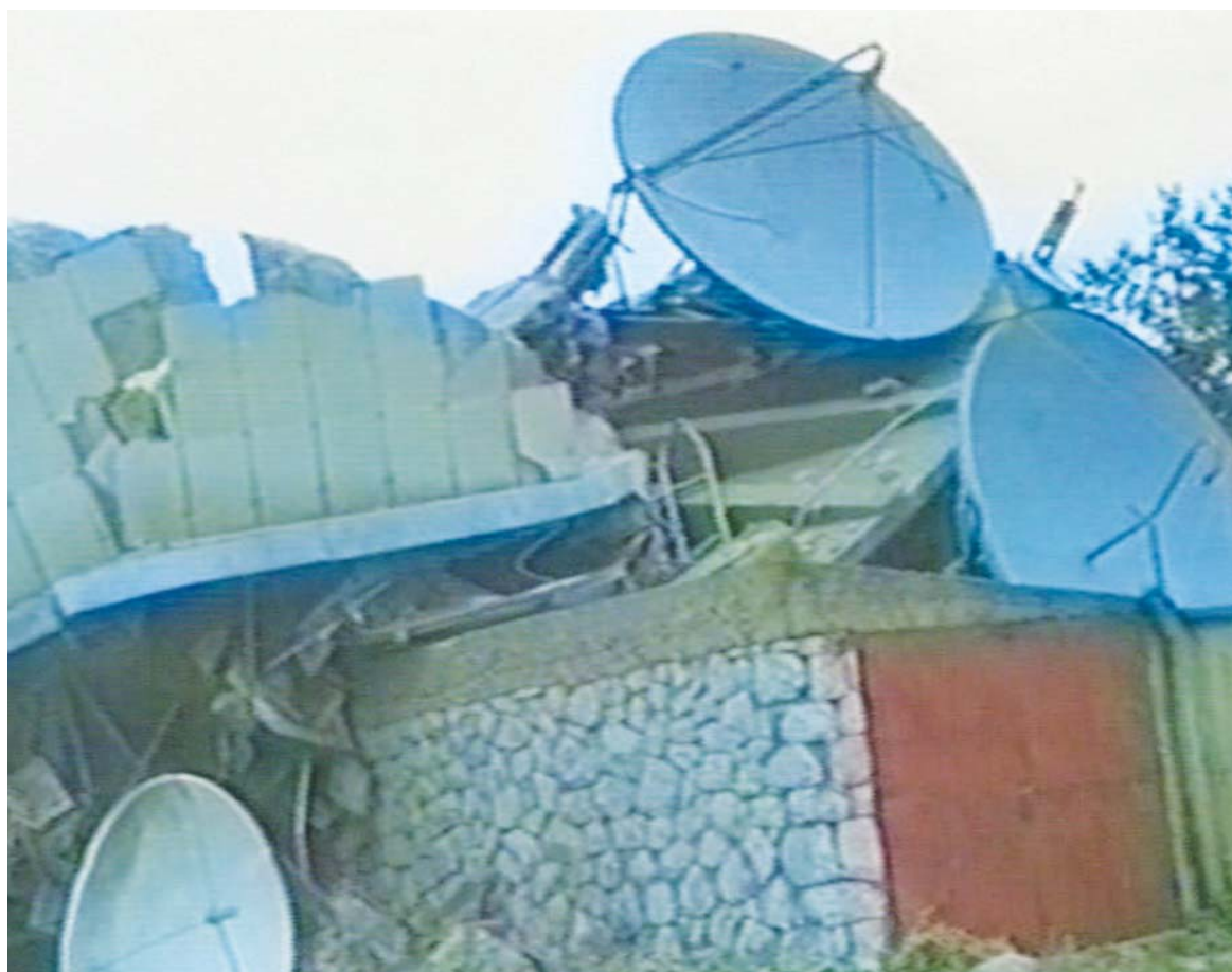
Picture 48. Destroyed radio-relay object on Lisina, Kozara
