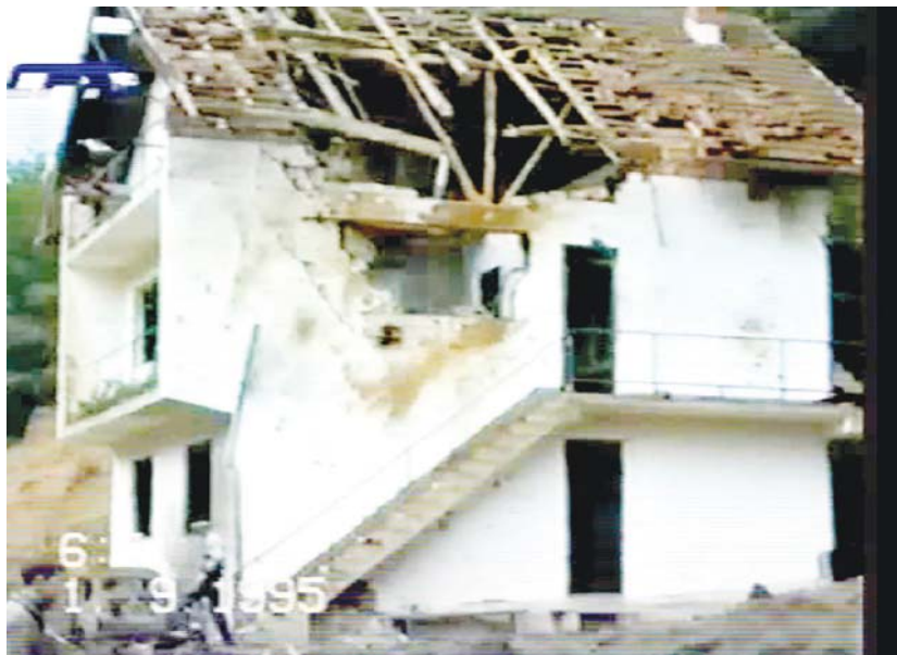
Picture 18. A destroyed residential facility in the area of Cajnice
