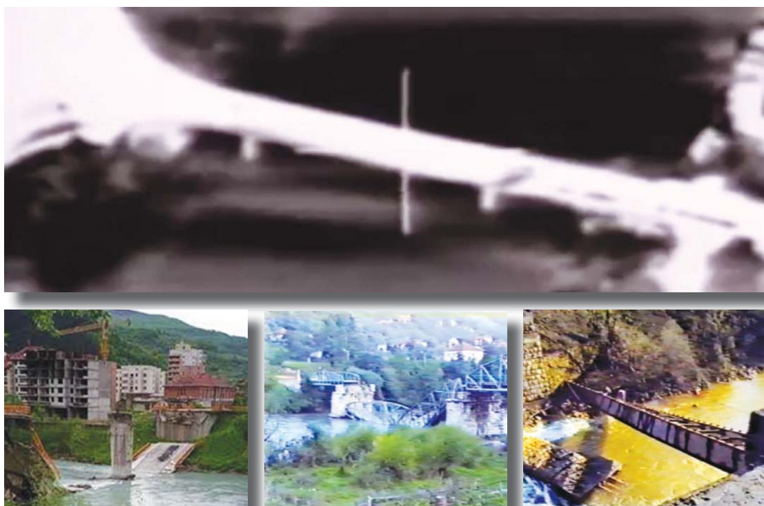
Picture 27. Destroyed bridges in the Municipality of Srbinje. In the pictures: aerial photograph of the US F15 just before firing the missiles (picture above) and the demolished bridges
