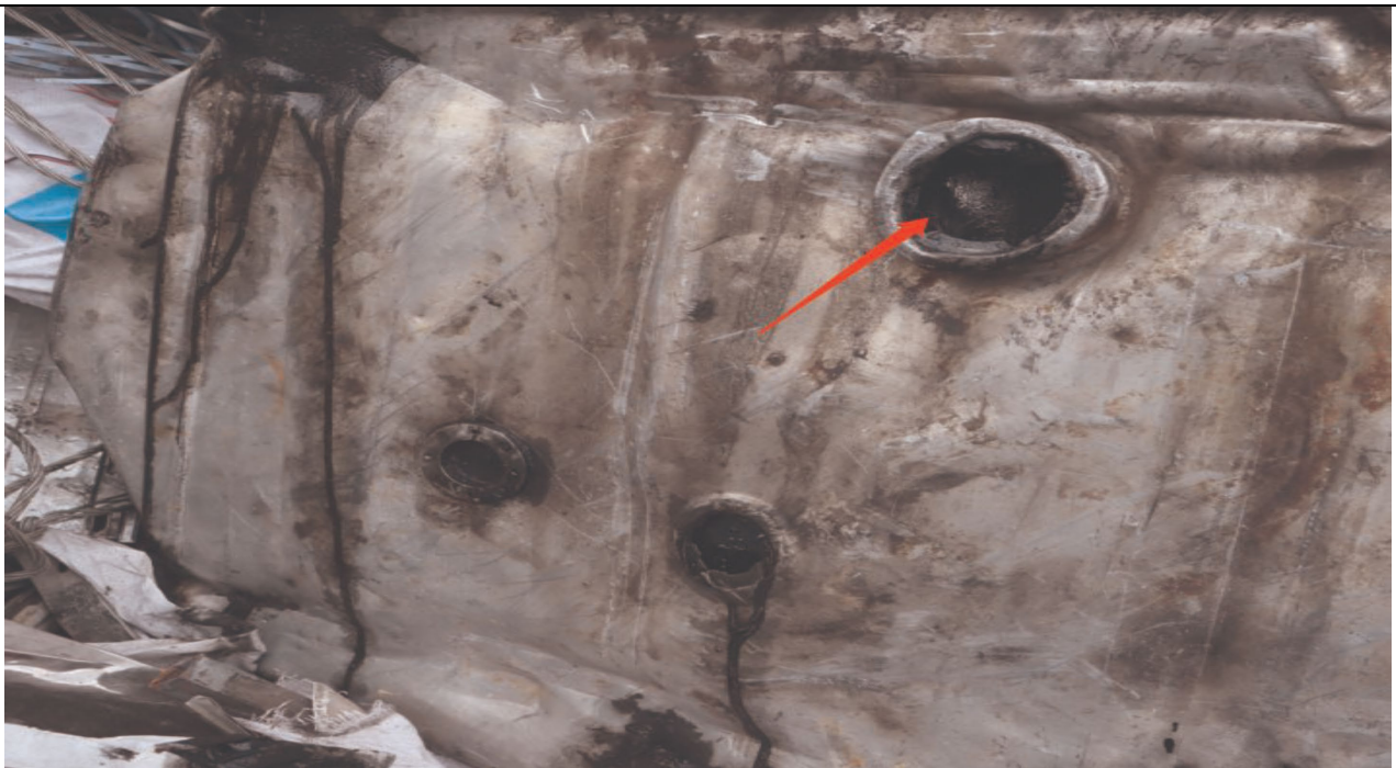
Figure A.13 Oil stains on aluminum appliances
