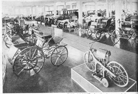
THE OLDEST: In the foreground is Gottlieb Daimler's two-wheeler of 1885 -the first motor-cycle in the world; next to it is the first Daimler car of 1886 and opposite are three Benz cars of 1896, 1897 and 1893 vintage respectively.
