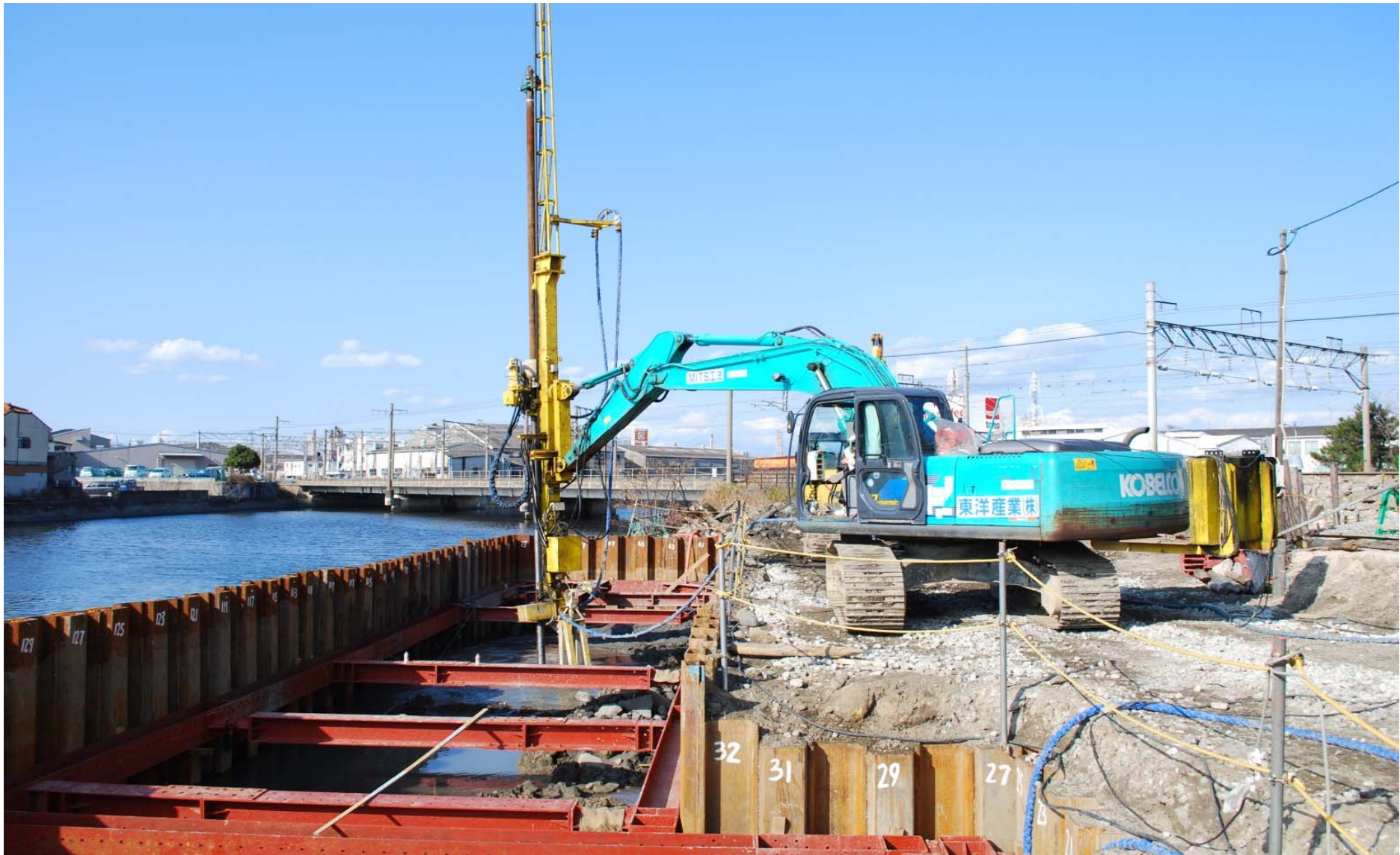
Foundation for Concrete Culvert Diameter \Phi 1600\text{mm} , Depth=2.4m
