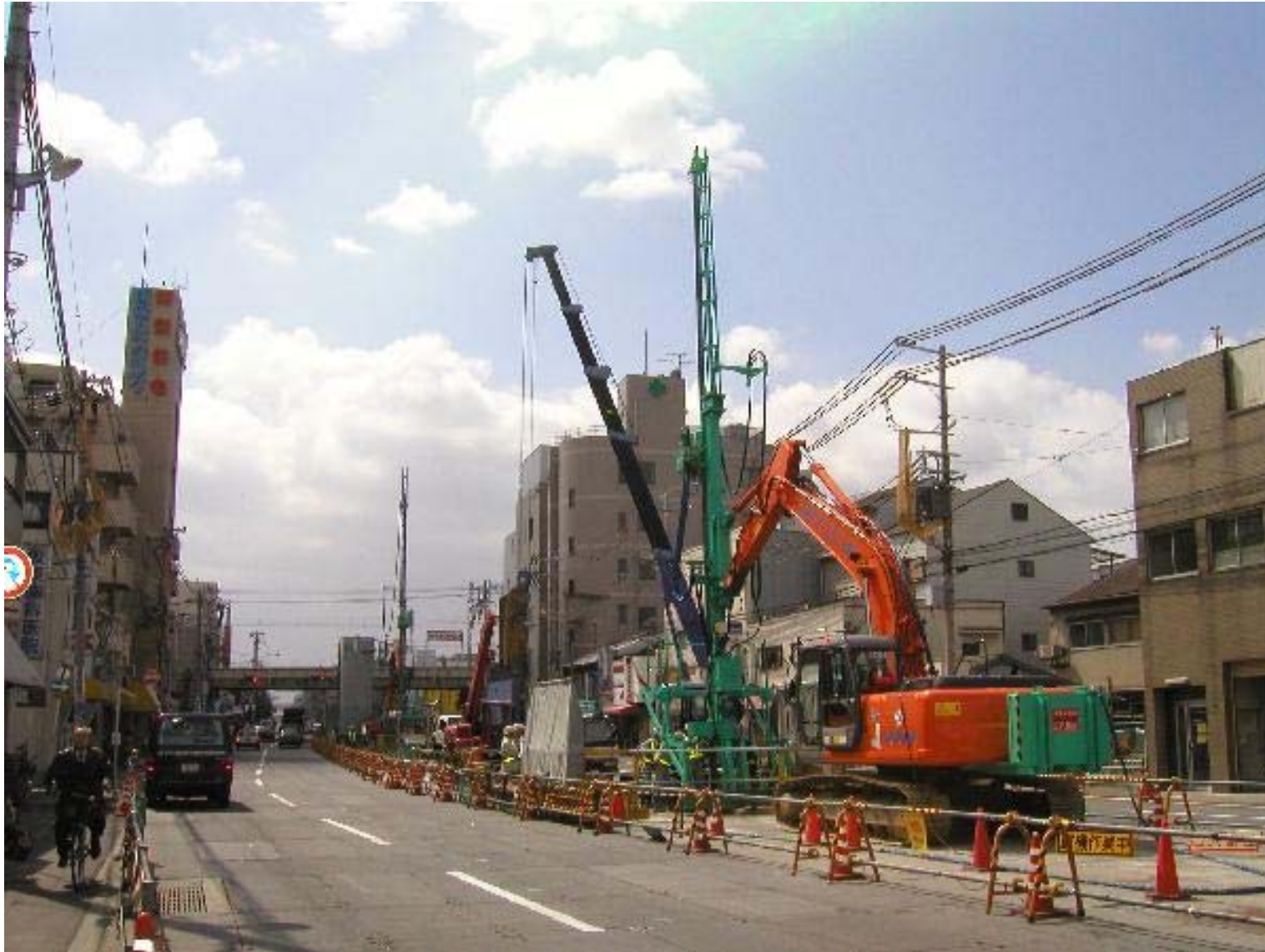
Subway Construction, Strengthen for soft ground Diameter \Phi 1400mm, Depth=16.0m
