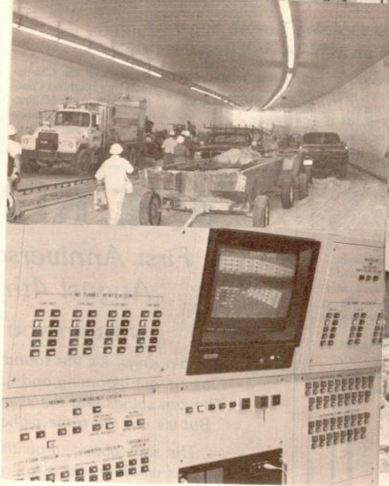
the Central Artery project . . . At the right is the CANA tunnel entrance from the Tobin Bridge, Route 1. BOTTOM ROW: At the left is the computerized tunnel emergency control system located underground in one of the CANA ventilation towers . . . On the right is a view
