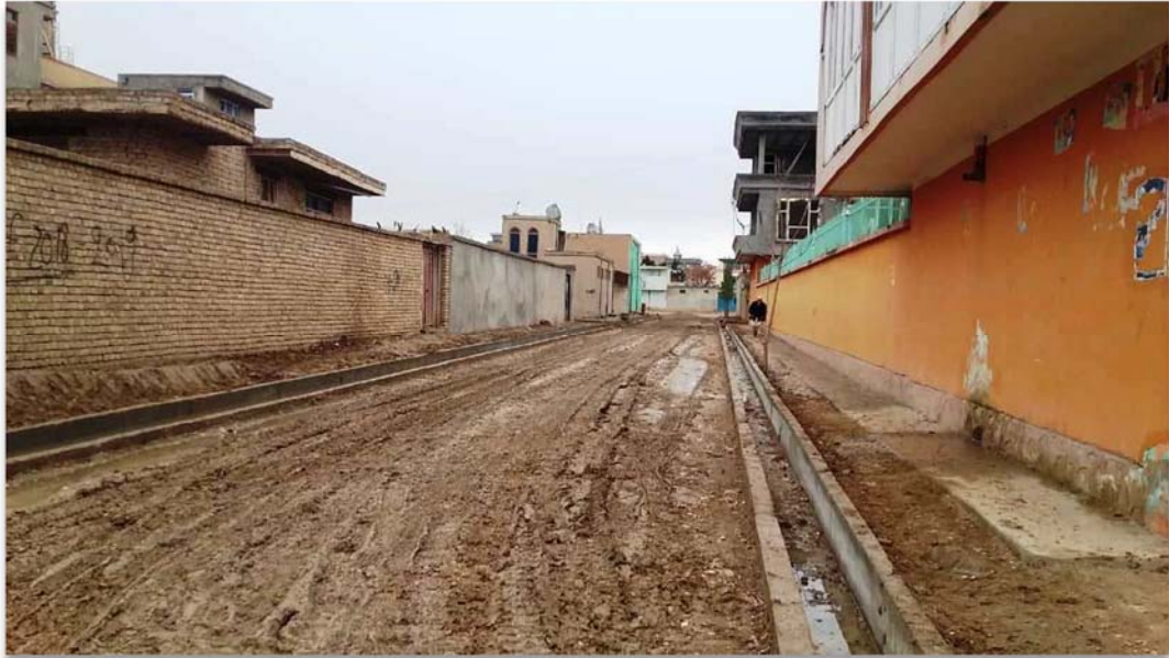
Rough streets under the process of construction
