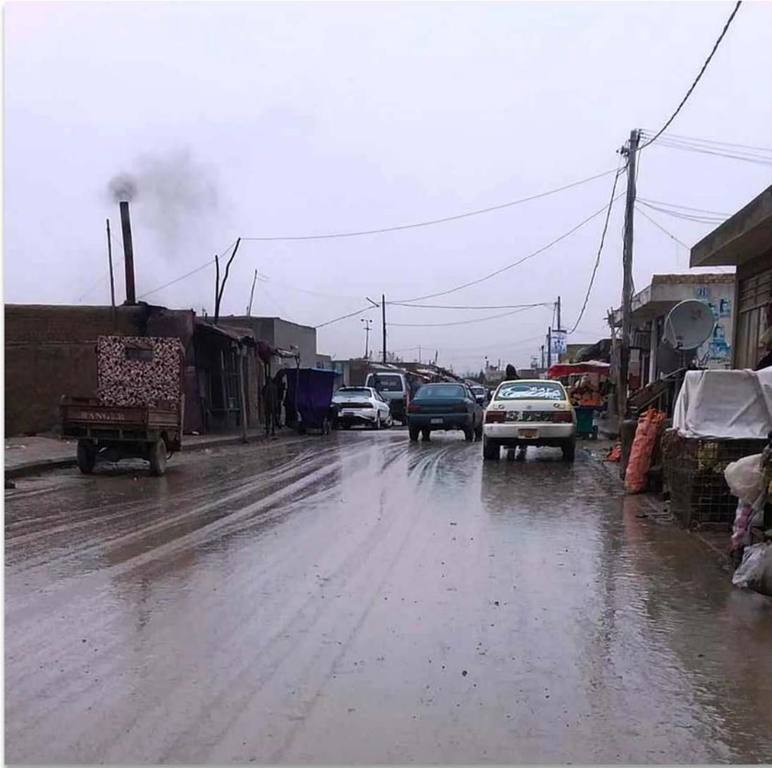
A click of main road constructed by support of Kadars
