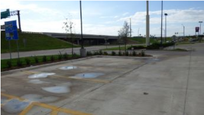
Front parking lot
