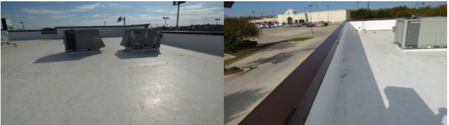
The roof is new and no recommended maintenance or repairs
