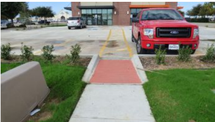
The parking lot is newly constructed with the handicap spaces, entry and exit signs, and parking spaced well marked.
