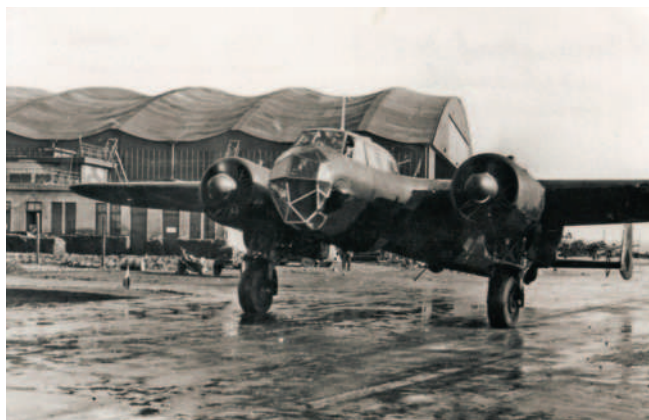
■ This aircraft of Küstenfliegergruppe 606 has had its undersides painted black for night operations. Again, the floatation bulges are clearly evident.
