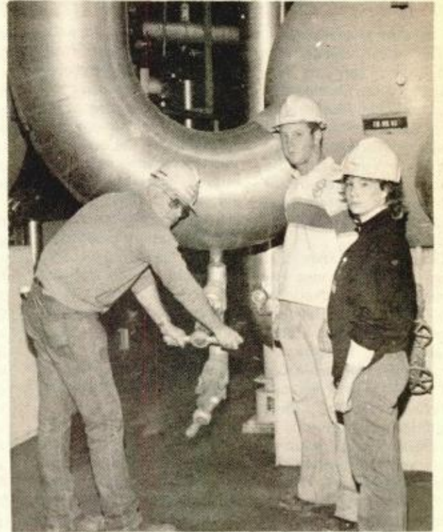
BOSTON EDISON's Peter McMahon (left) demonstrates how to close a heater drain backstop at the company's Mystic 7 steam plant. With him are Massachusetts Maritime Academy cadets Michael Walsh of South Boston and Dawn Dineen of Charlestown.
