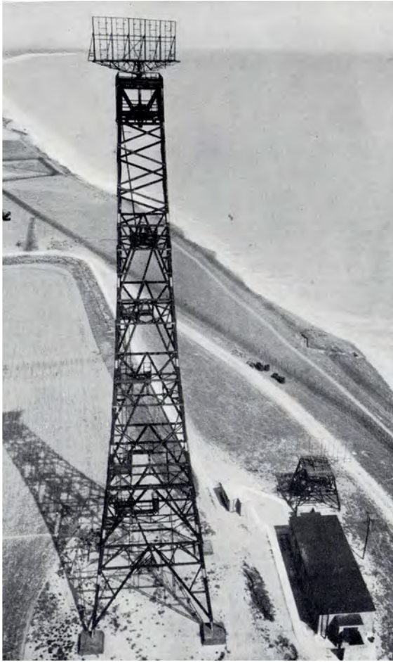
ABOVE A Chain Home Low (CH(L)) radar tower, a development of Watson Watt's Radar concept aimed at detecting aircraft flying at low levels.
