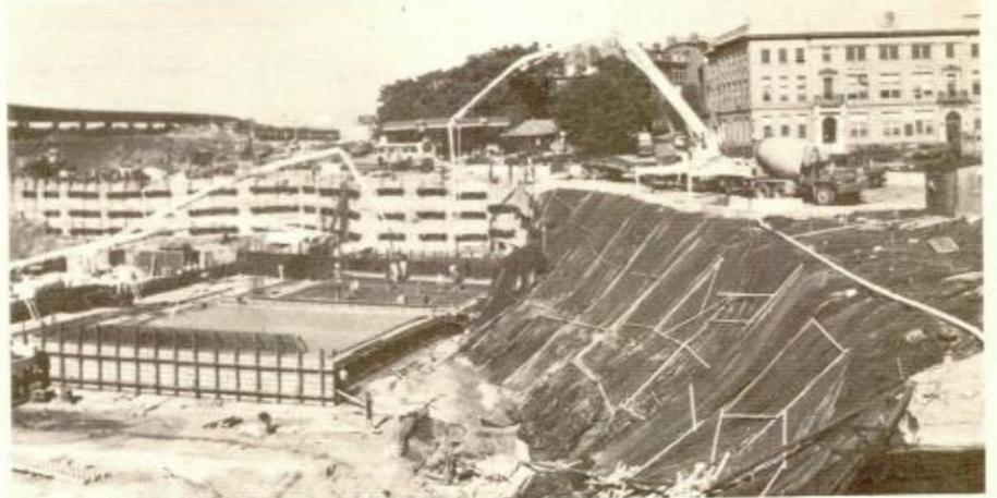
THE CEMENT FLOOR of the southern portion of the tunnel is being poured where the former Y.M.C.A. building once stood. One of only two landmarks left in City Square, the Charlestown Courthouse, is seen at right of photo.
