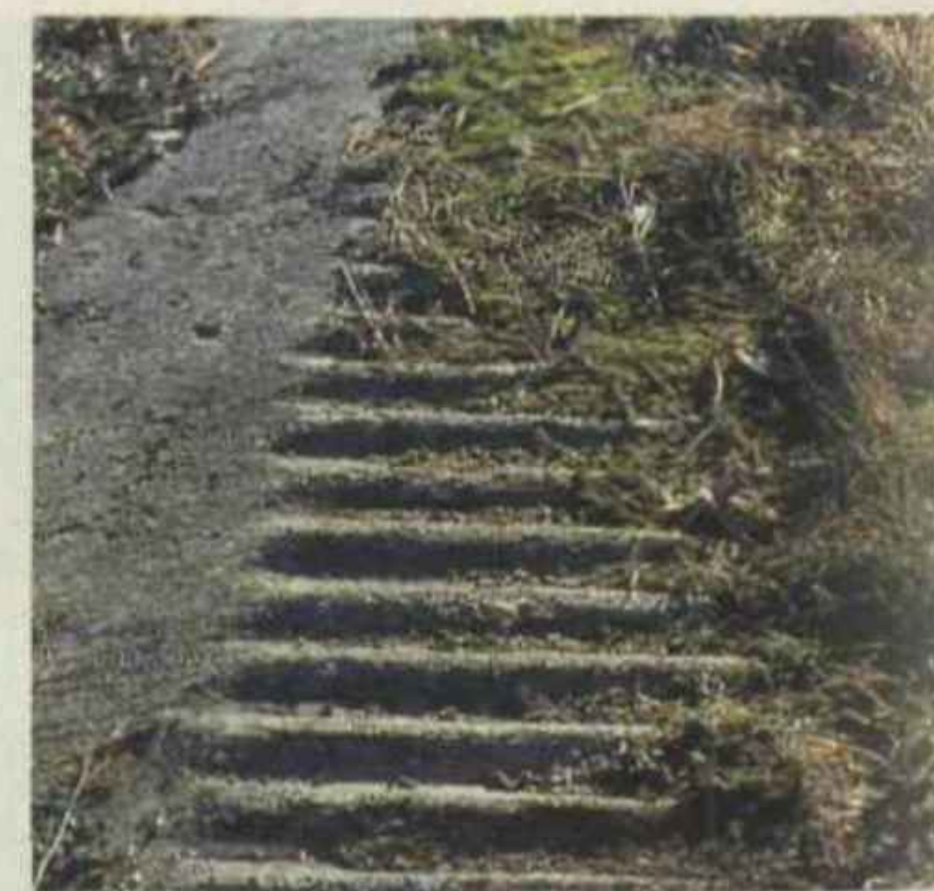
All that remains of the old track... Crumbling rumble-strip at Masta
