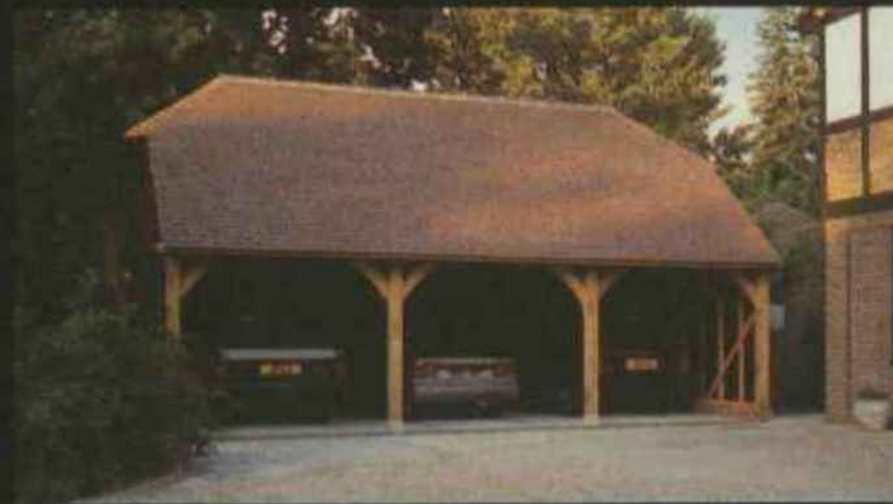
THREE BAY GARAGE No. 180
