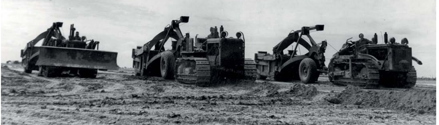
Three bulldozers and scrapers, working in echelon, level the area to be used in the construction of a new, all-weather hard runway at B.10/Plumetot airfield, in July 1944. RAF (AHB)/© UK MoD Crown Copyright 2014
