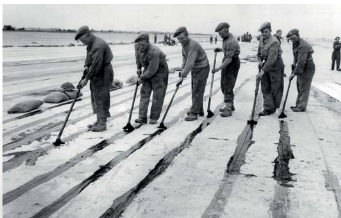
Right: Men of the Pioneer Corps, an army unit providing labour for light engineering tasks, caulk PBS during construction of the hard runway at B.10/Plumetot airfield. A 'fairweather strip' was located off to the left. RAF (AHB)/© UK MoD Crown Copyright 2014
