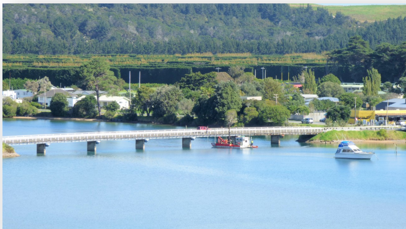
Taipā bridge with a sediment survey boat at work beneath it.
