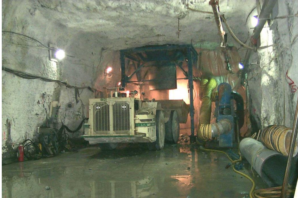
Photo 4 Ore Collection Chute below a Production Raise
