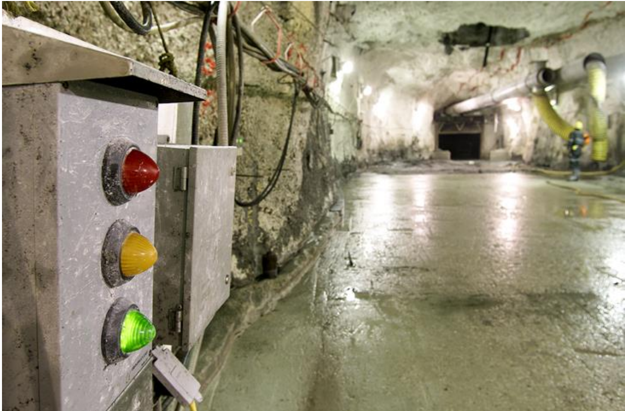
Photo 7 A Radon Progeny Monitor in a Typical Raisebore Extraction Chamber
