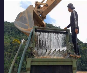
Cristian, Excavator Op.
