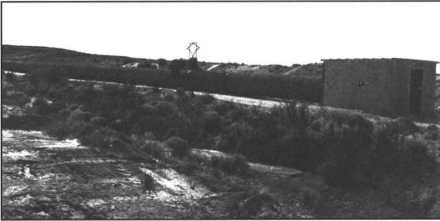
Figure E-1 - Tunnel Range showing exposed pipe before covering with earth.
