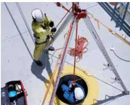
Tripod as High Directional System
