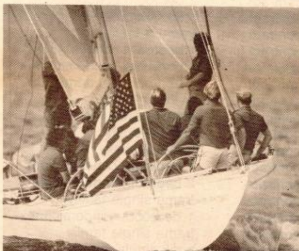
COURAGEOUS II, training in waters off the coast of Bermuda, for its quest to recapture the prized America's Cup from Australia in 1987. The 12-Meter was redesigned to include an innovative, aerospace-inspired Vortex Wing keel developed by Leonard Greene, chairman of The Courageous Challenge.
