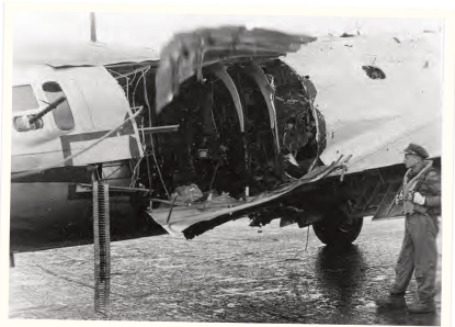
ABOVE: A direct hit by a heavy flak shell was almost always lethal, although B-17G 42-98004 of the 508th BS/351st BG had a lucky escape. During a raid on Cologne on September 27, 1944, an 88mm shell entered the fuselage near the rear entrance to the radio room and blasted away the ball turret. It made it back to the 351st BG's base at Polebrook, Northamptonshire, where its pilot, Capt Jerome Geiger, was photographed surveying the damage
