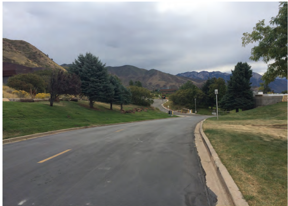
View to east along access road.
