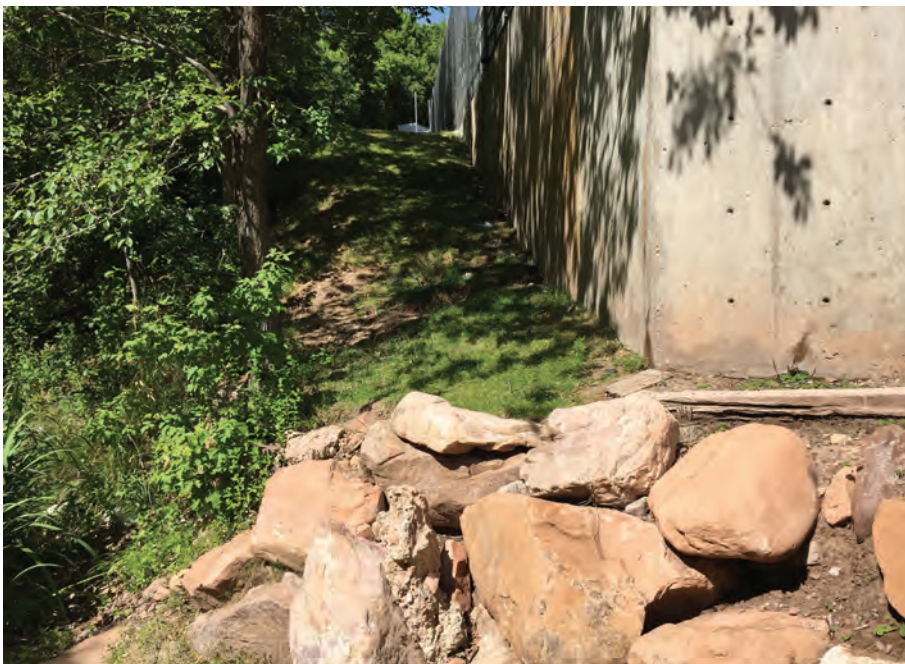
Narrow area of passage between retaining wall and streambanks.
