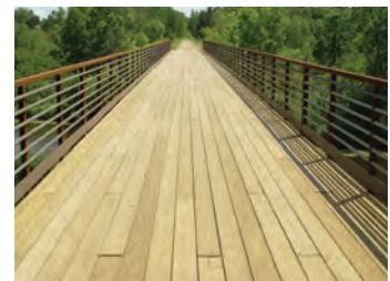
Example of bridge with visual access.
