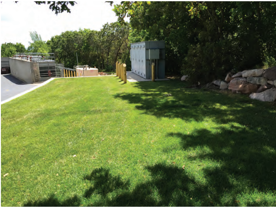
View of utilities located along buildings northwest corner.
