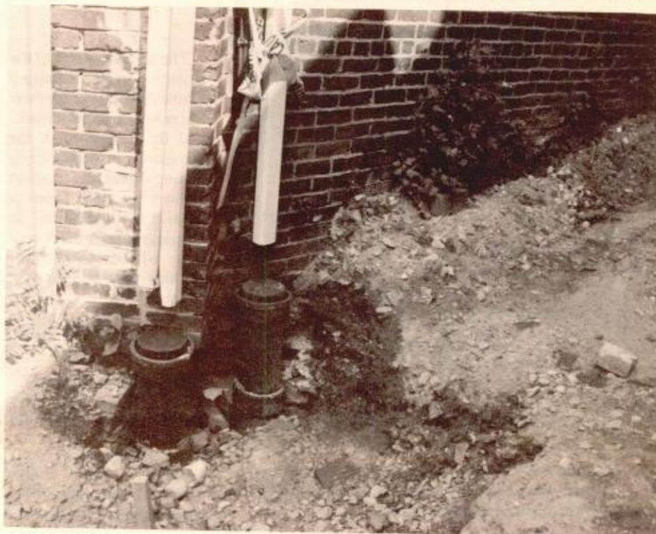
A BROKEN FOUNDATION of a house on basement. Common Street allows water to enter the
