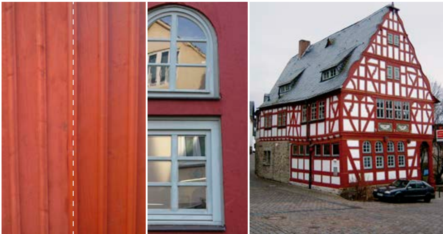
| One coat finish after 15 years of aging | After being freshened up with a single coat | Red and grey are often a very attractive combination | The old town hall in Niederbrechen, Germany
