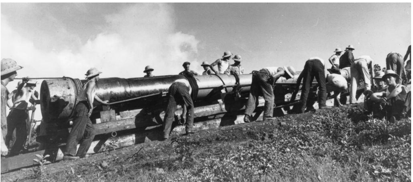
The eight guns were installed in pairs in four batteries placed on high ridges at four corners of the island. Moving the barrels uphill was somewhat eased by the fact that much of the vege-
