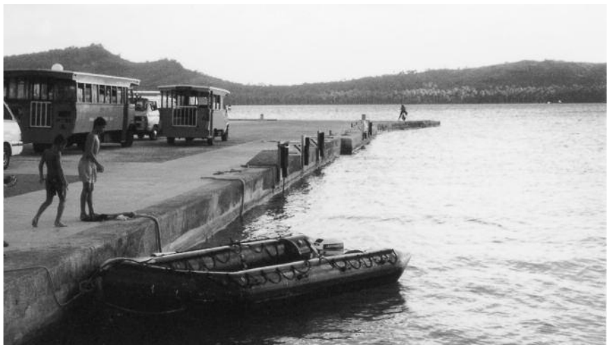
A much larger concrete dock was built by the US Navy's 1st Construction Battalion — the original Seabees — soon after their arrival. Today, this is used by air passengers who are shuttled by boat to and from the airport on nearby Motu Mute.
