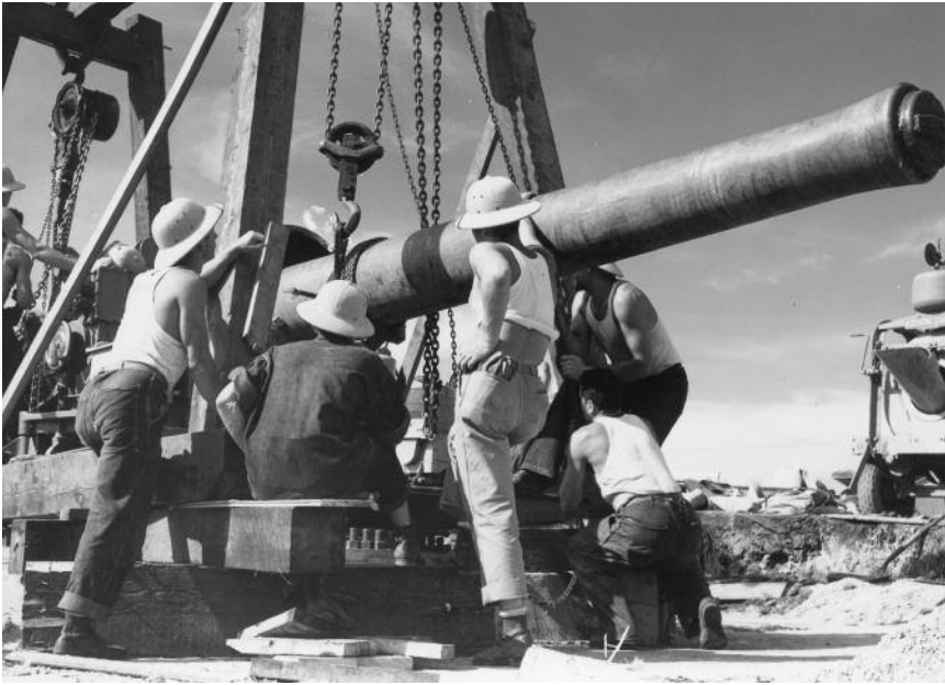
The Americans mounted eight 7-inch guns on the island. These came from the old battleship USS Connecticut which had been scrapped in 1923. Installation of the 28-ton guns was a difficult job, requiring much ingenuity, improvisation, and sweat. Here, one of the barrels is lifted using an A-frame. (US Navy)
