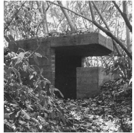
The battery's fire-control bunker.
