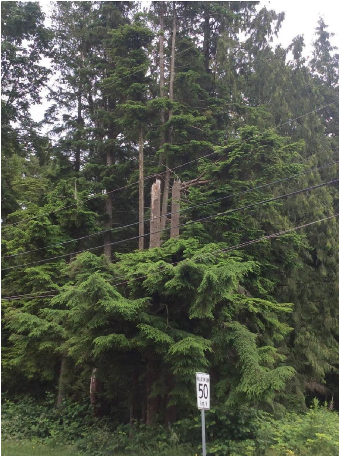
Figure 4. Stem breakage along the road near hydro lines along McCombs Ave and adjacent to the East Sector lands.
