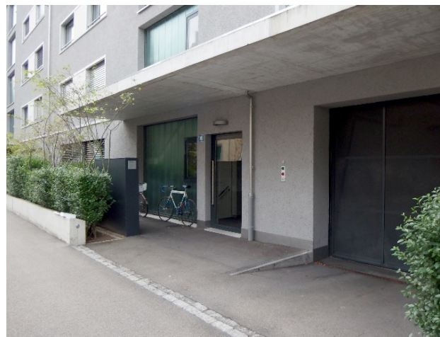
Reference Goldbrunnenstrasse Zürich, compact parking entrance integrated with the main house entrance (image vdw)
