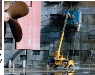
Repair of a dry dock wall. Dubai, UAE.
