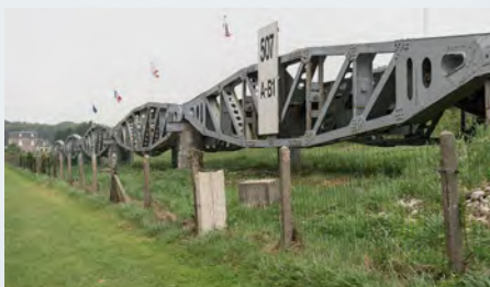
ABOVE: The Invasion of Normandy was kept supplied by these Mulberry Harbours designed for the rapid offloading of cargo onto the beaches
