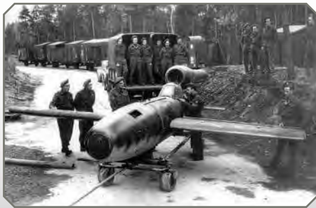
The Fieseler Fi 103R Reichenberg was a manned version of the V-1 'Doodlebug' flying bomb and designed as a suicide bomber. It was never used in anger
