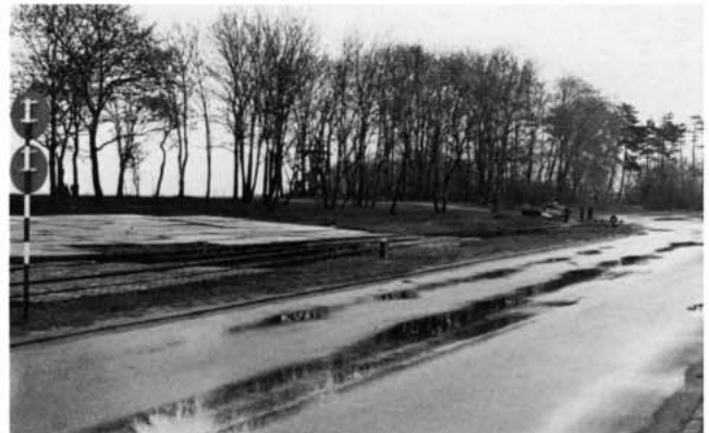
The station building survived almost intact up to the sixth day when it was blown up by German pioneers. Right: The attack came up the track on the right, the gate being situated roughly where the group of posts now stand.
