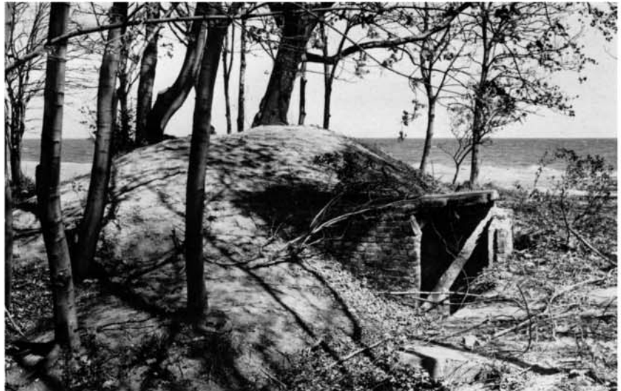
The emplacement just north of the railway, about 200 metres behind the station, from which Corporal Edmund Szamlewski and two men with a light machine gun decimated the initial German attack.
