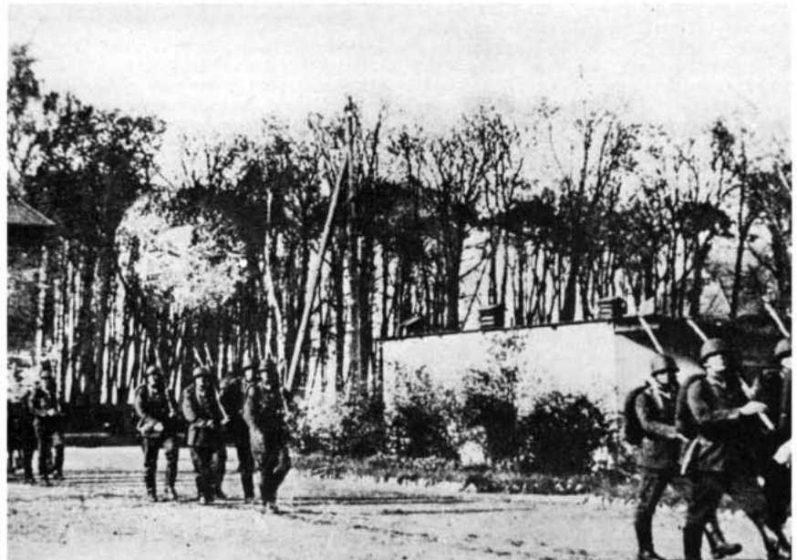
Mounting the guard in 1939. On the left is the old barracks.
