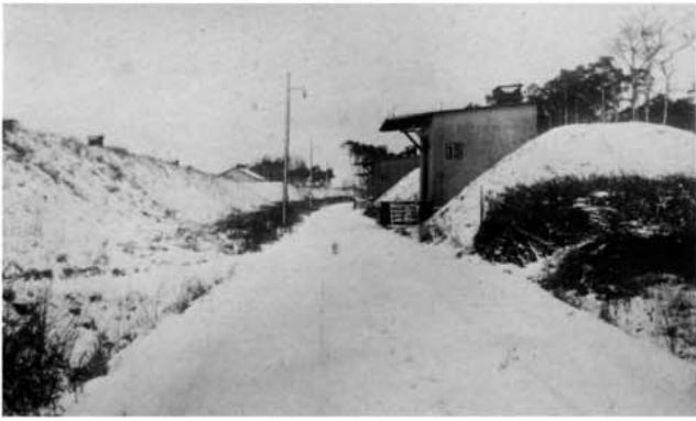
Earth embankments protected the ammunition storage shelters — these three being situated beside the railway track on the north-eastern perimeter facing the sea (see map overleaf).
