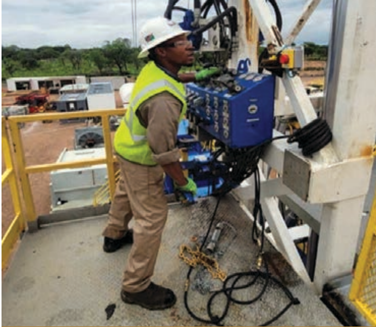
At the end of December 2020, 44 personnel are currently on-site, of which 39 are Namibians. Of the 39 Namibians, seven are from the Kawe Village nearby where ReconAfrica is completing test well drilling for conventional oil.
