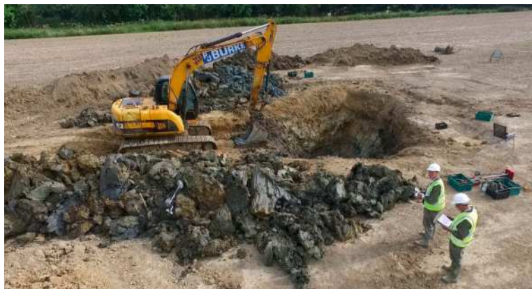
■ A wider view of the Marden excavation in 2019.
