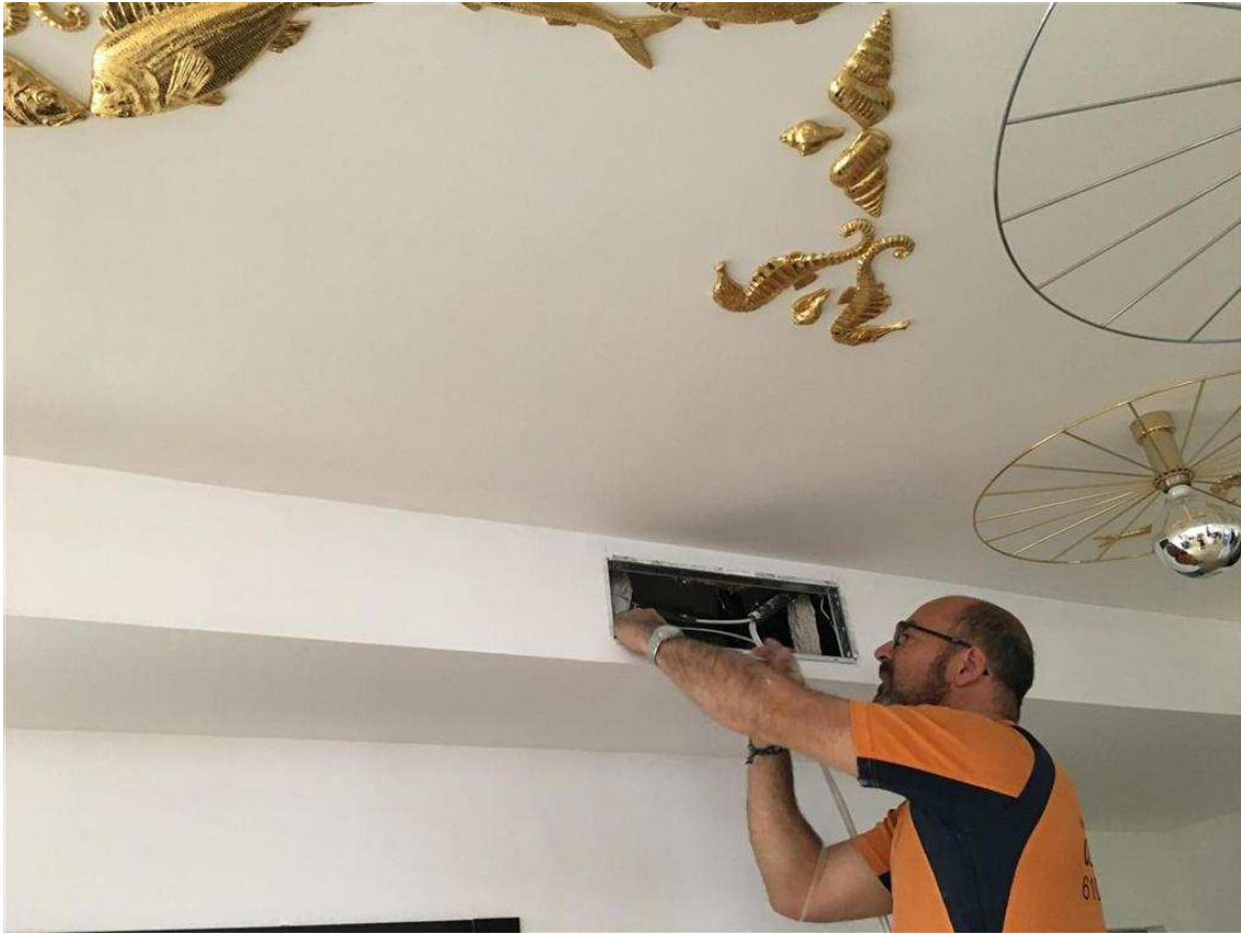
Looking for the best way to run the cables!
