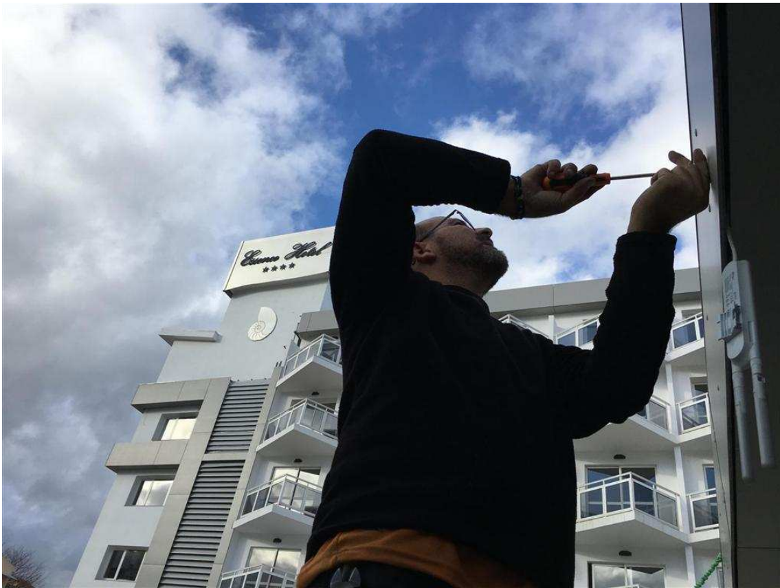
UAP AC-M install.
