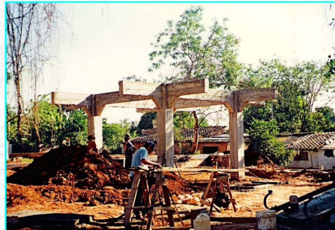
Construction of the Base: Treatment Plants
