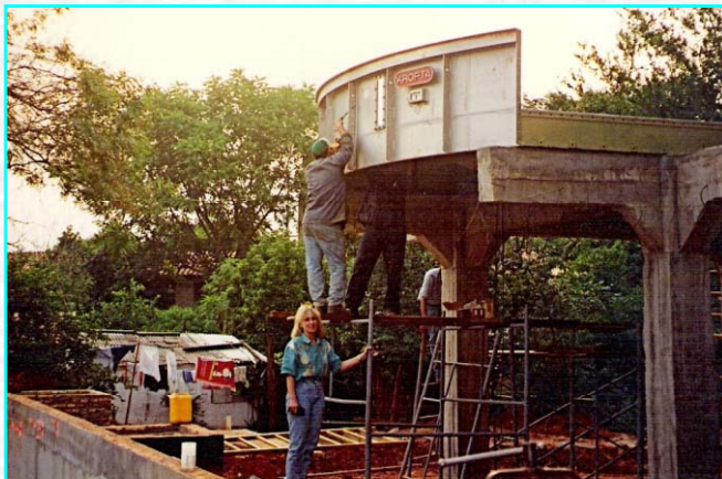
Controlling the Construction Work in Lambaré
