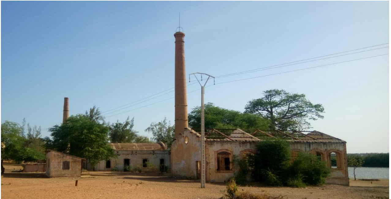
Figure 5: Current view of the old Makhana factories
