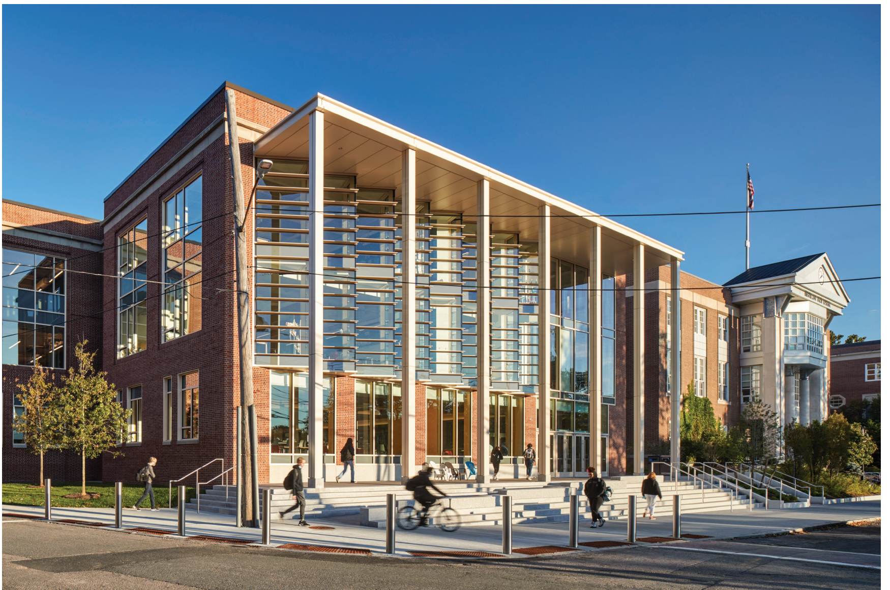
STEM wing addition to Brookline High School, designed by William Rawn Associates. ROBERT BENSON
