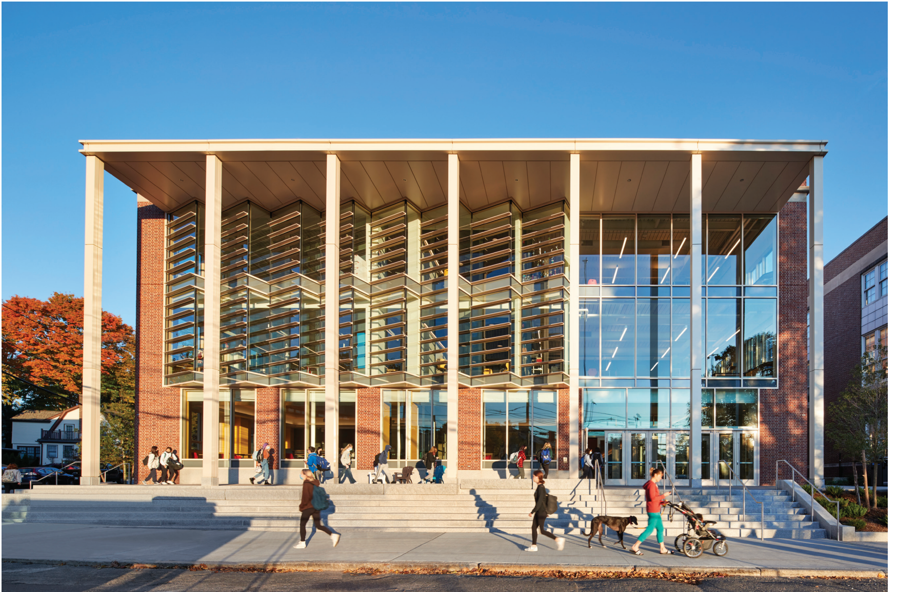
STEM wing addition to Brookline High School, designed by William Rawn Associates. ROBERT BENSON
