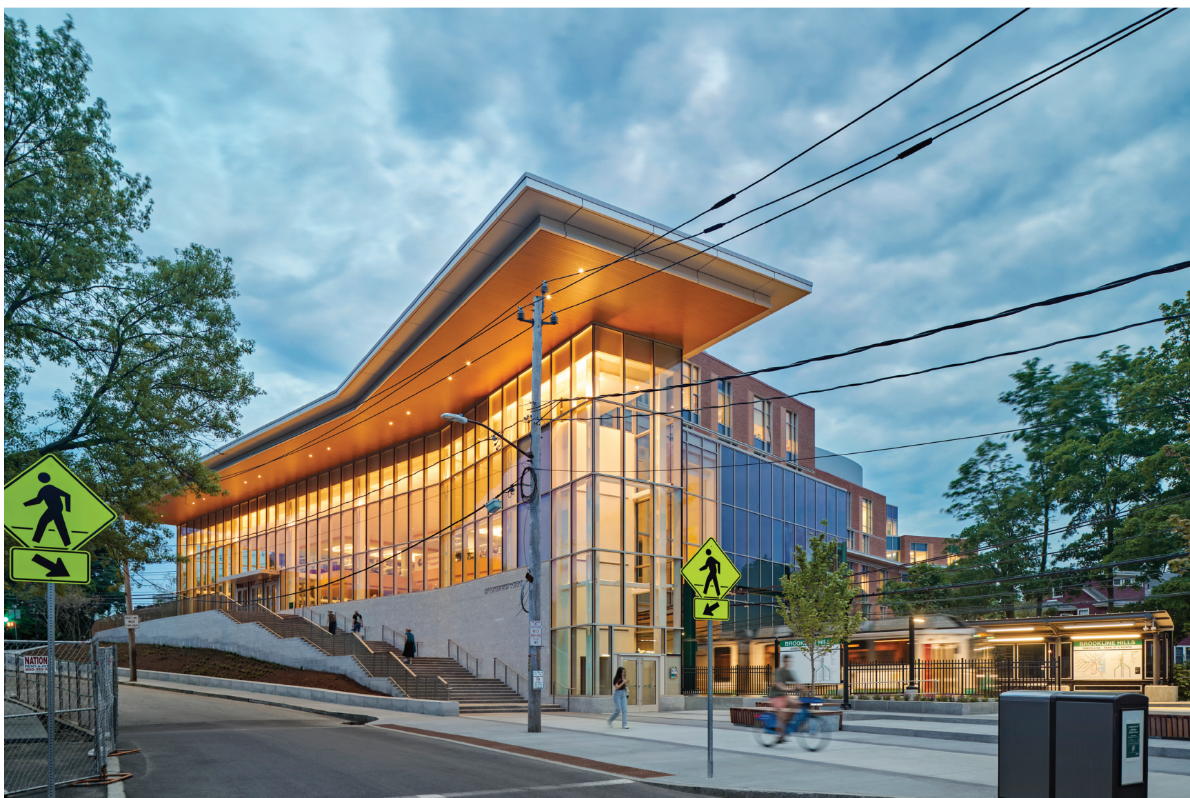
Brookline High School's 22 Tappan Building, designed by William Rawn Associates. ROBERT BENSON
